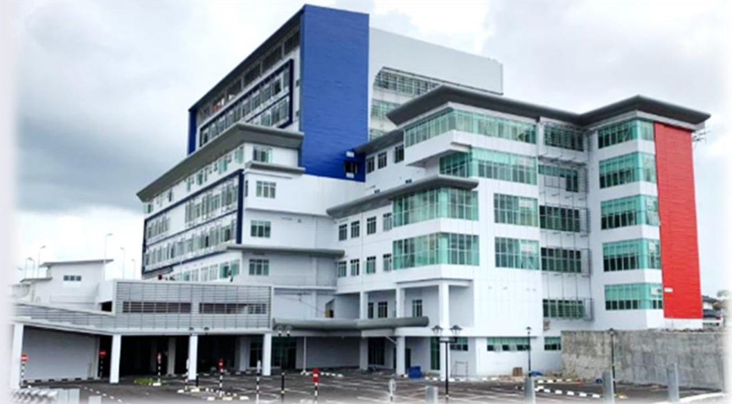
BDC Kuching - relocation
